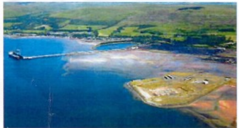
Hunterston Port and Resource Centre (PARC)
